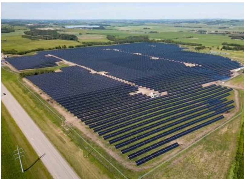
Elemental Energy Inc. Innisfail Solar Farm
