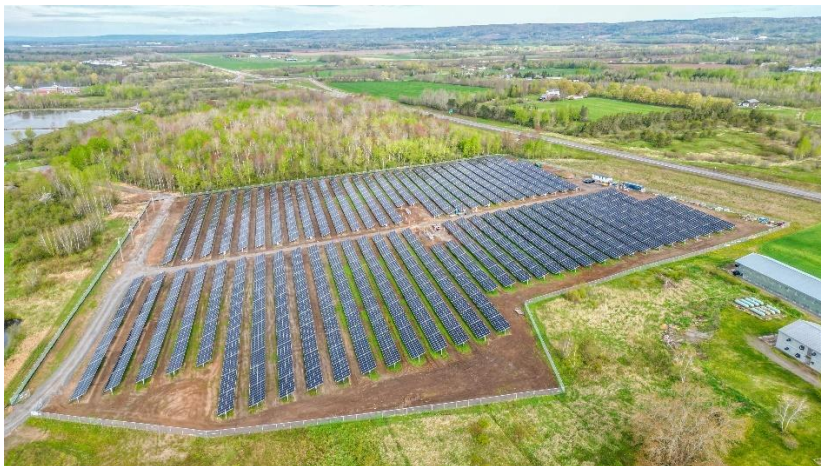
Berwick Solar Farm
