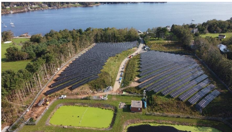
Mahone Bay Solar Farm
